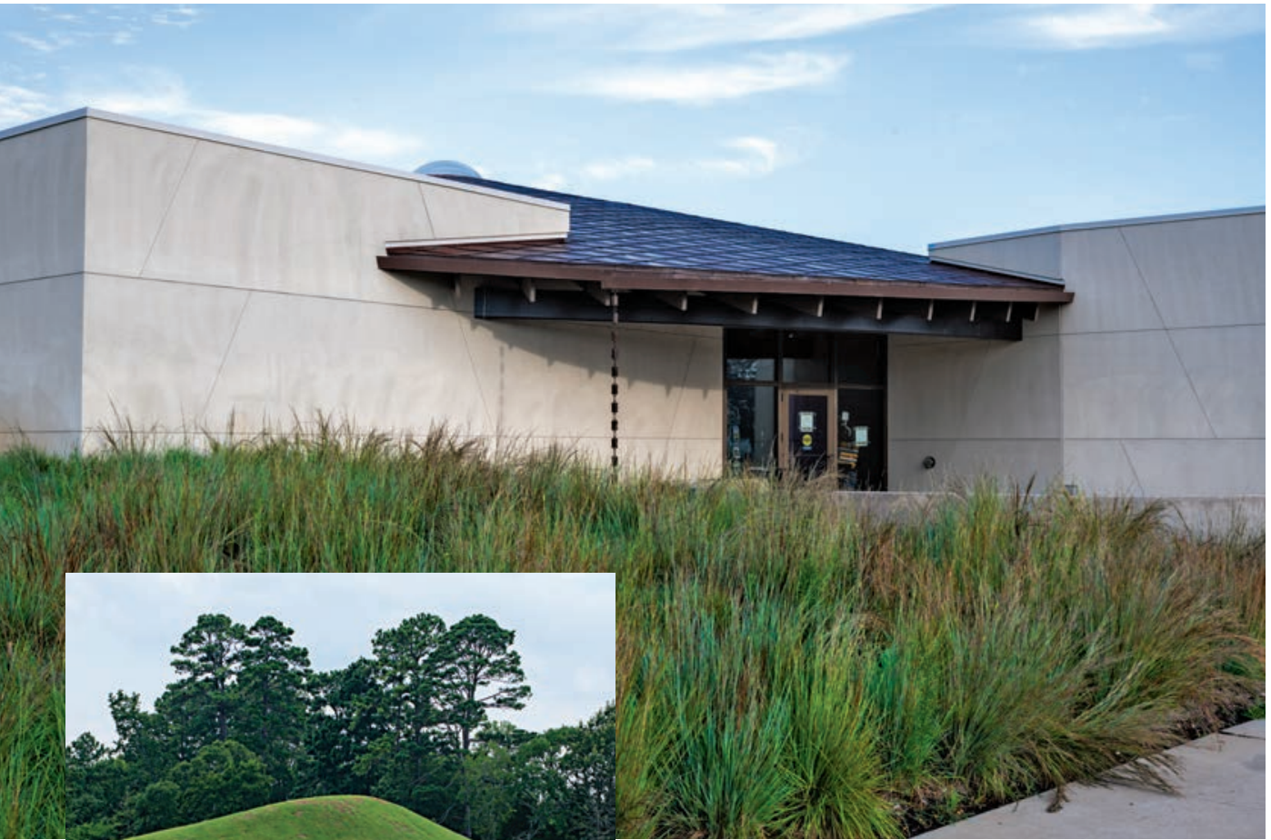
ABOVE The exterior of the new visitor center was designed to blend into the natural environment with a self-weathering steel roof intended to mirror the shape of the Caddo mounds.
